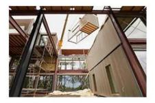
The building structure is calculated and verified with CYPE software taking into account the connection existing among different modules which make up the whole structure.
